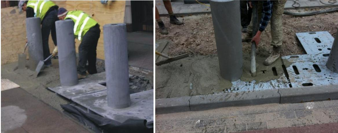
The concrete should be poured flush with top plates and biscuits and clear of excess concrete.
